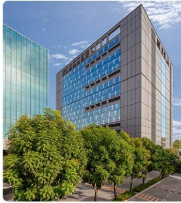
Gigaplex IT Park - Building 9, Mumbai
