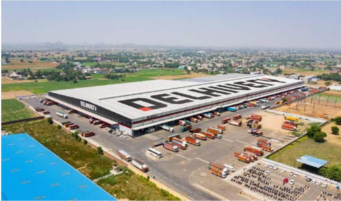
Aerial View of the Tauru Gateway (Haryana)
